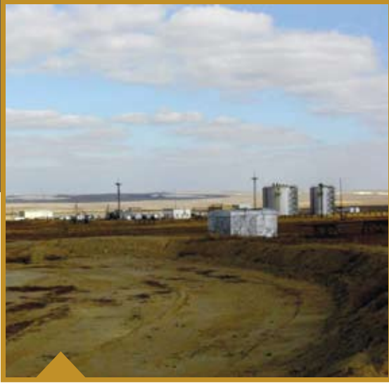
Laktibay Storage Tanks / Kazakhstan
