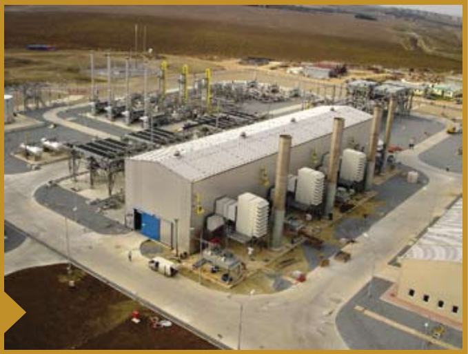
Silivri Natural Gas Storage Facilities
