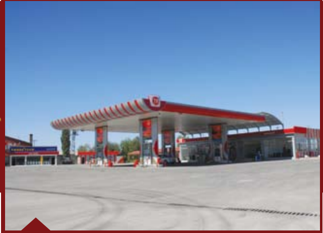
TPPD Fuel Station
