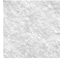
Figure 12. The defective tile image for Crack defect
